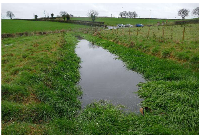
1 st swale at Farm 2 showing strong grass growth within the swale
