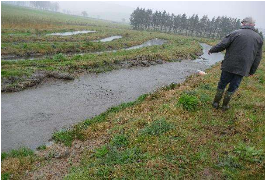
Swale System at Farm 5 showing excessive presence of slurry solids in the first swale that the system was not designed to handle and also surface flow of dirty water seeping from a swale bank to the river.
