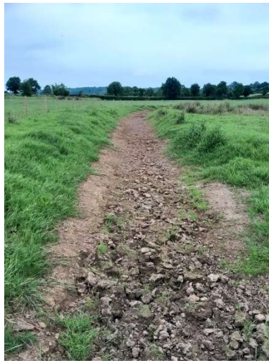
Photo 9: Pebble swale under construction 2
