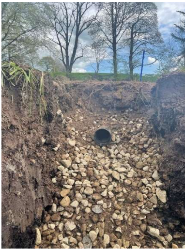
Photo 10: Pebble swale under construction 1
