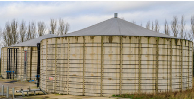
Figure 6: Fixed cover on an above-ground concrete slurry store at CAFRE.
