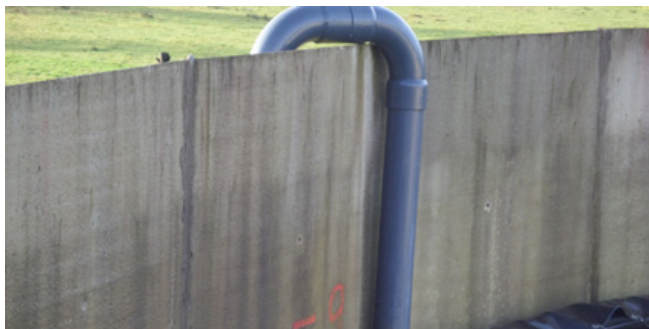
Figure 8: Detail of tank fill pipe. Note that the tank fill pipe is extended down the inside of the tank to facilitate filling from the bottom when a floating cover is installed.
