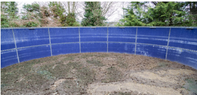
Figure 10: Slurry tank with crust which can help to prevent ammonia loss.
