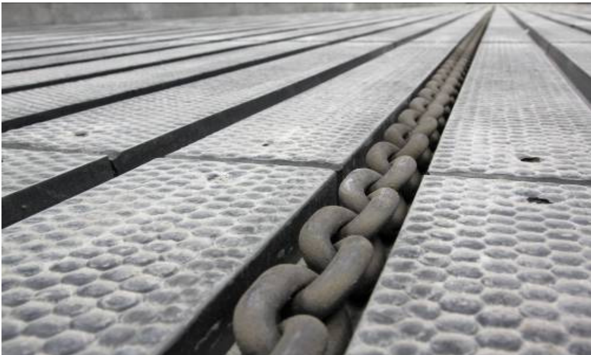
Rubber grooved floor installed either side of the feed passage in the Cafre dairy unit
