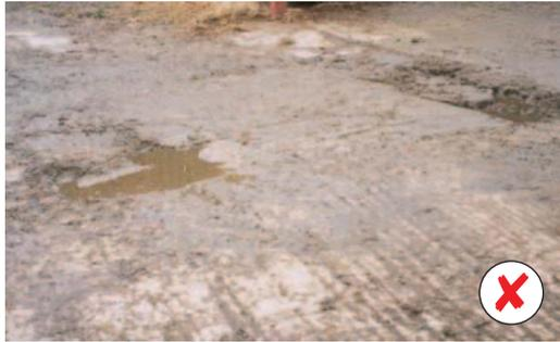
**Fig 9a** Avoid potholes in worn concrete which can cause lameness and damage to feet
