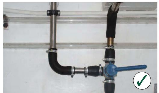
**Fig 11** Valves fitted to divert circulation wash to the footbath after cleaning milk plant
