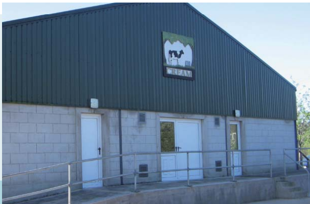
ABOVE LEFT A purpose built facility houses the 30 strong Creamer herd.
